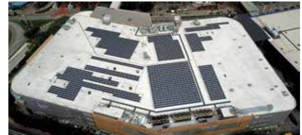
Ikano Power Centre (IPC) Shopping Mall Reroofing, Mutiara Damansara, Selangor
