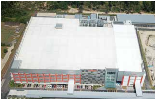
Osram Opto Semi Conductors, Penang (Malaysia)
