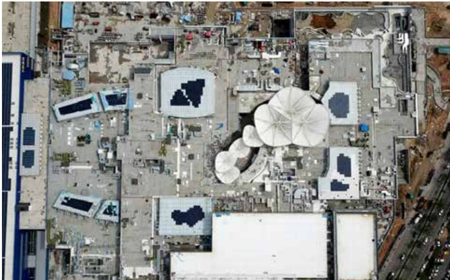
Ikano Toppen Shopping Centre, Johor Bahru (Malaysia)
