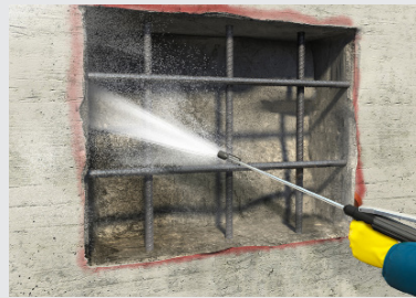
Substrate and Steel Preparation
