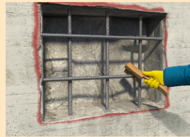
Application of Repair Mortar
