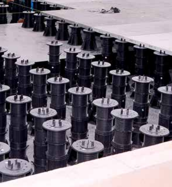
Pavers laid directly on pedestals
