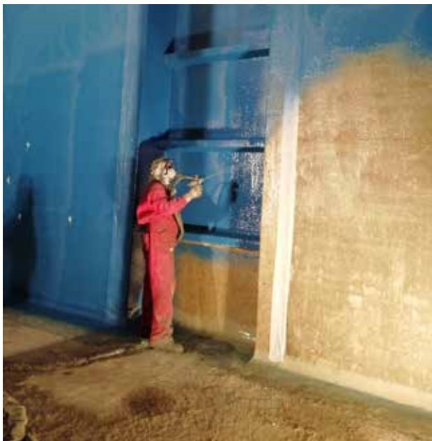
Reservoir Santa Cruz del Valle, Spain: 1,800 m 2 of Sikafloor®-161, Sikalastic®-840 ES.
