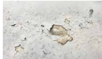
Existing liquid applied membrane
