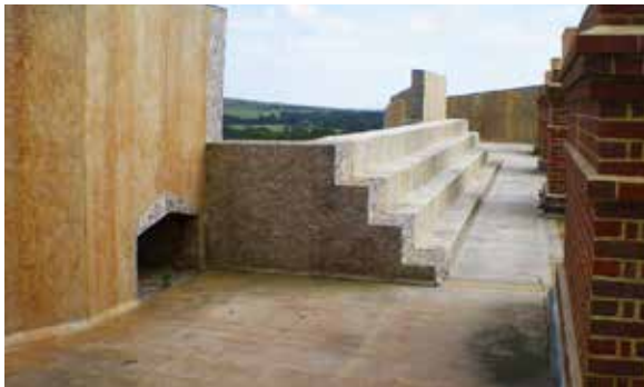
BRICKS AND STONES
