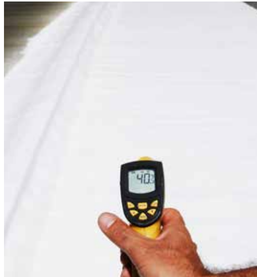
Roof temperature after LAM application.
