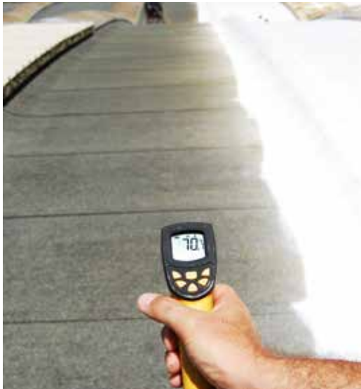
Roof temperature before LAM application.
