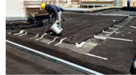
Torch on bitumen membrane
