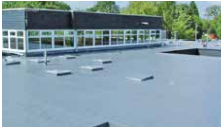
Exposed concrete roof
