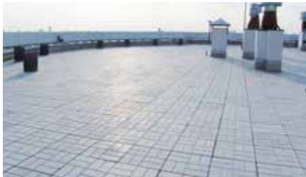
Concealed concrete roof
