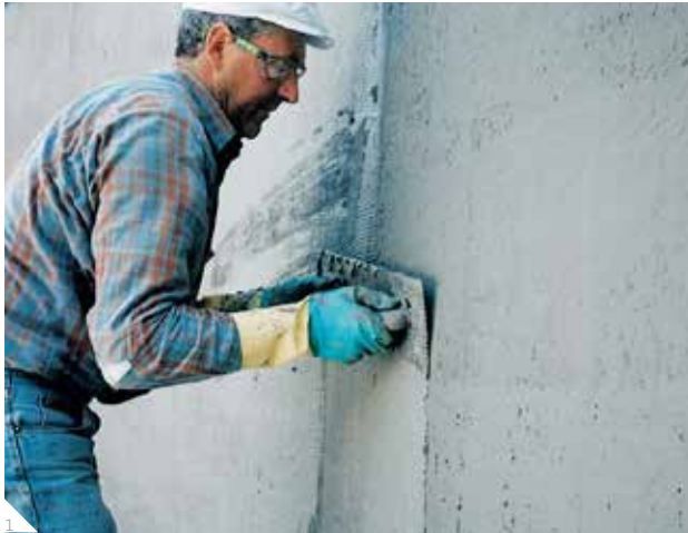
1 Waterproofing mortars and renderings
