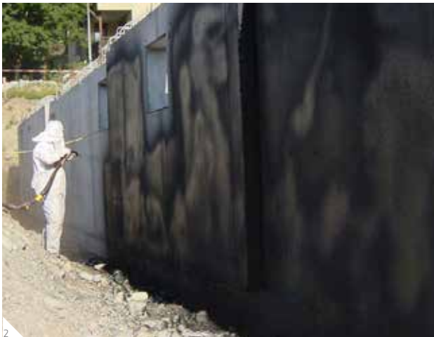
2 Bitumen coatings
