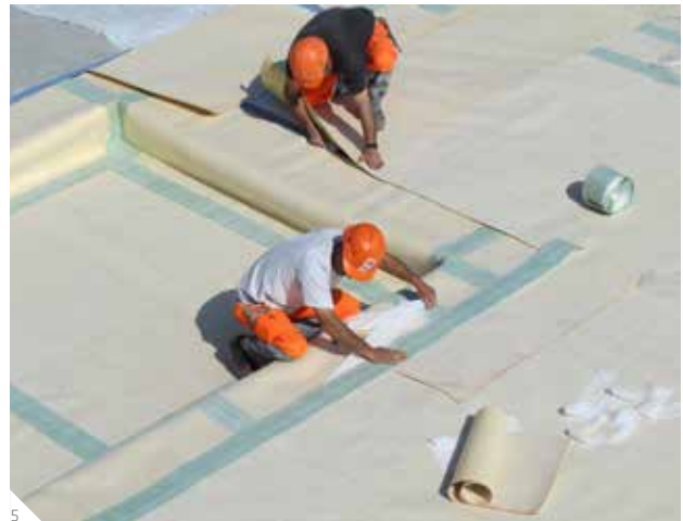
5 Fully bonded sheet membranes
