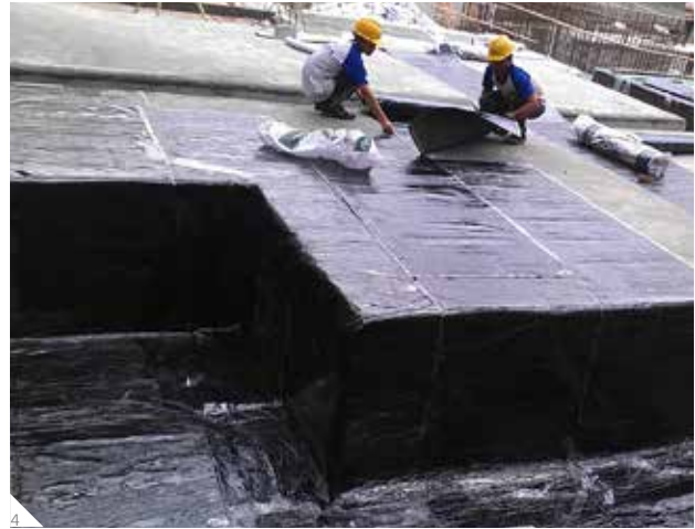
4 Wet bonded sheet membranes
