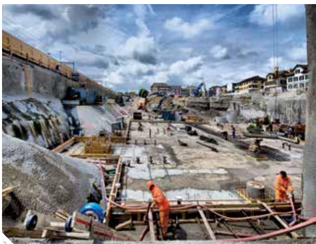
3 Sika White Box concept/Watertight concrete
