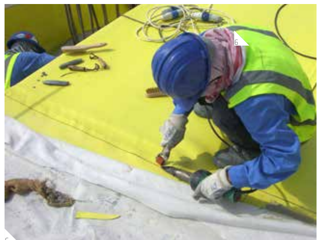
6 Compartmentalized sheet membrane systems
