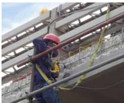
Substrate preparation
