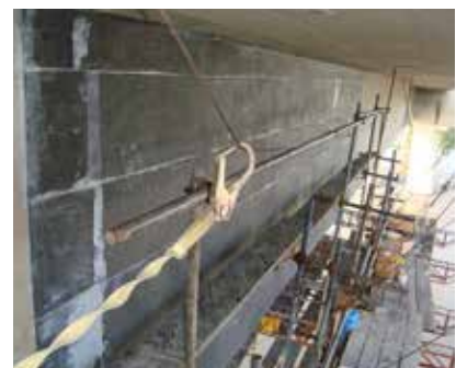
Strengthening with SikaWrap®
