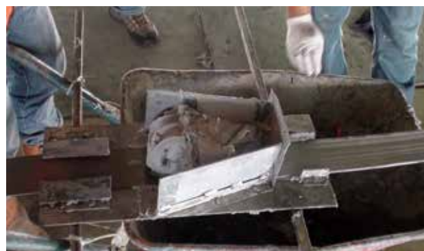
Coating of CarboDur® plates with Sikadur®
