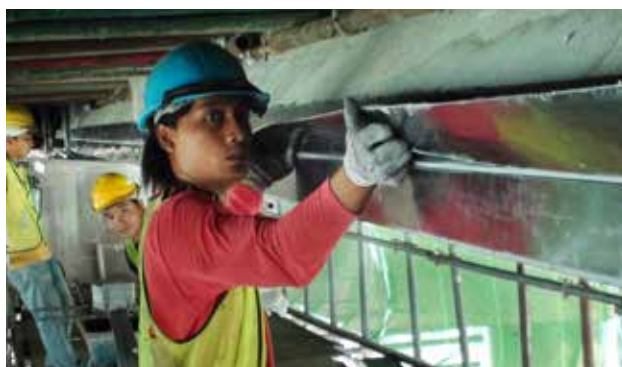
Installation CarboDur®
