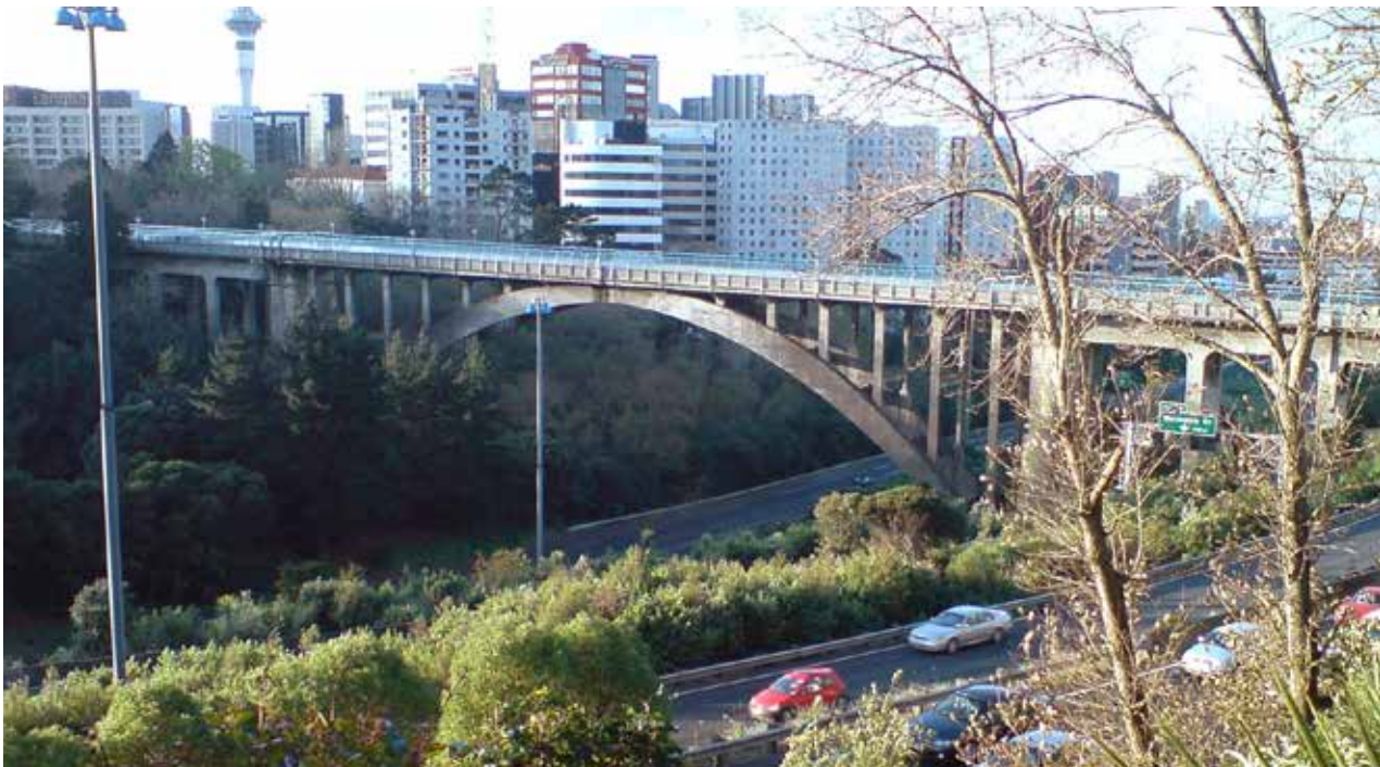
Grafton Bridge, Auckland, New Zealand
