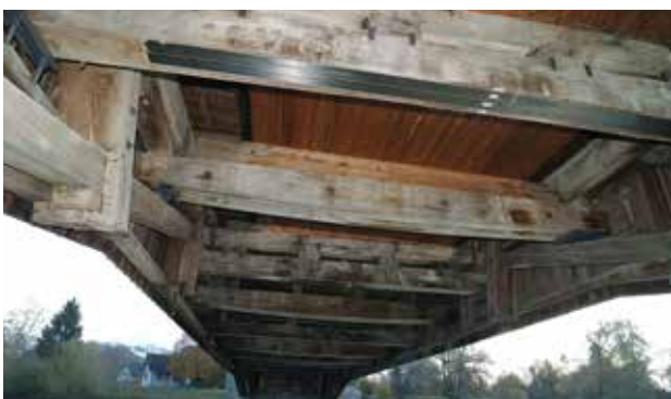
CarboDur® strengthened crossbeam
