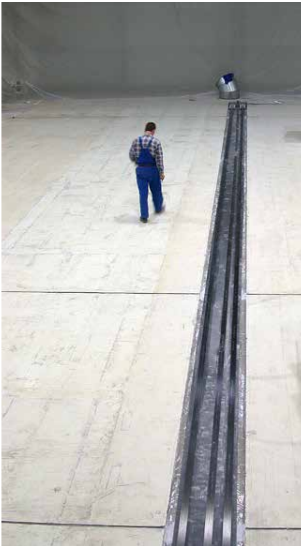
The longest post-tensioned CFRP-plates ever installed
