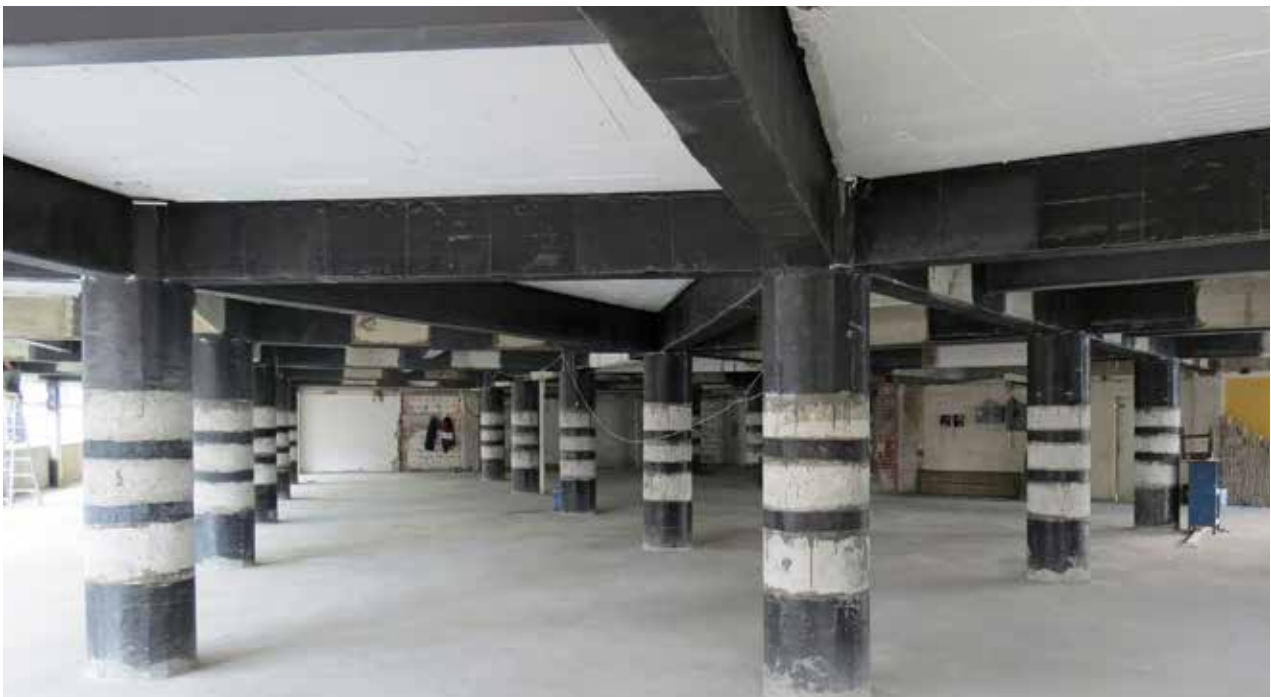
Beams and columns strengthened with SikaWrap®
