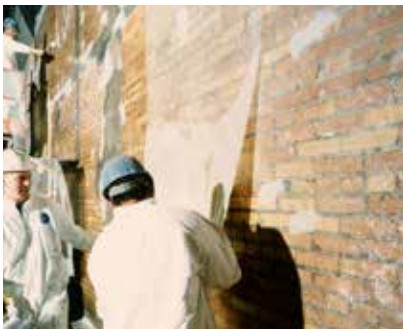
SEISMIC UPGRADING /EARTHQUAKE DAMAGE REPAIR
