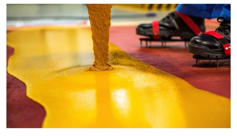
Sika provides liquid applied floor finishes and cementitious underlayments to protect, prepare, upgrade and finalize floor surfaces. Our full range of seamless flooring solutions meet the highest requirements for both industrial and decorative floor systems. We use a wide range of technologies such as cement, calcium sulphate, epoxy, polyurethane, hybrid versions among others.
