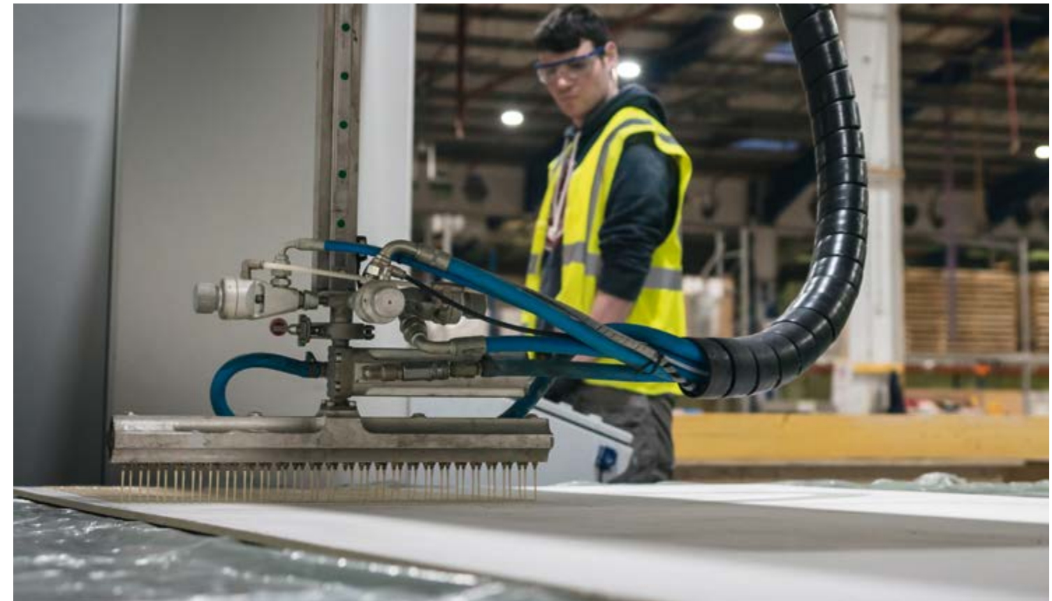
SikaForce® applied by spreader bar
