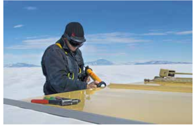
Once the flat roof panels were installed, the pre-painted panels were then sealed with SikaHyflex®-250 and layered with wooden battens to replicate the Hut's original appearance.
